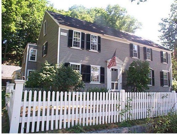
Thomas Dane House, 47 Lexington Road, ca. 1650. Perhaps the oldest remaining house on Lexington Road, it retains some First Period architectural characteristics, including massing in the steeply-pitched roof and one-room-deep arrangement of its main section. Enlargements and alterations occurred in the 18th C. One of the oldest houses in Concord.
