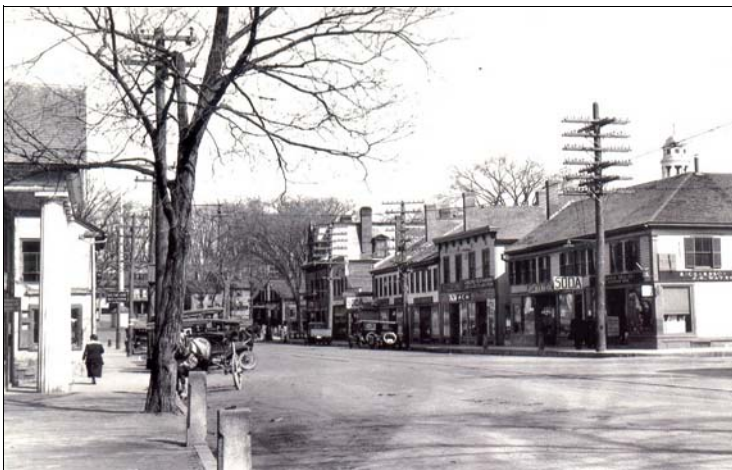
The Mill Dam from the north-west, March 31, 1921 Main Street Historic District. Photographer: Herbert Wendell Gleason
