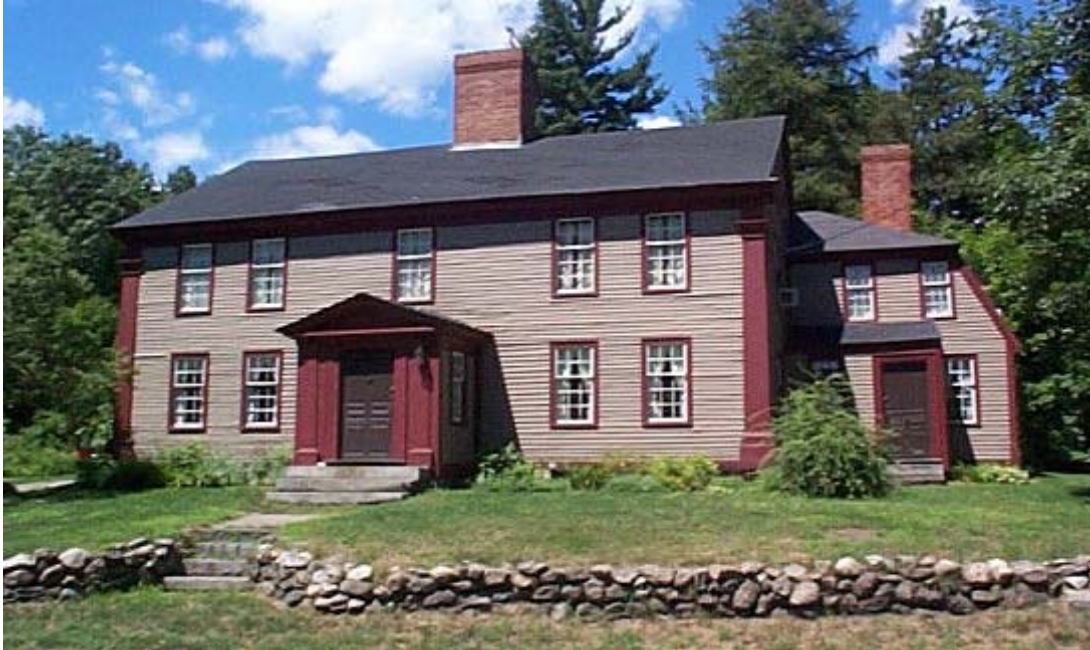
572 Main Street, Joseph Hosmer House, ca. 1672, Main Street Historic District. The core of the structure is a First Period house, the home of Obadiah Wheeler, an original Concord settler. Major Joseph Hosmer, a well-known cabinet maker and farmer, probably added the rear portion and gambrel ell ca. 1757. The house retains many important early features and decoration. One of the oldest houses in Concord.
