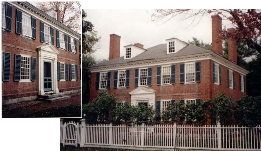
8 Barrett's Mill Road, Jonathan Hildreth House, 1750. Barrett Farm Historic District. Eminently important as one of Concord's finest examples of high-style late Georgian architecture at the point of transition to the Federal style. It is the town's only large brick house of the style, and an outstanding illustration of the work of master builder Reuben Duren. (Concord Survey of Historical and Architectural Resources, Vol. 1)
