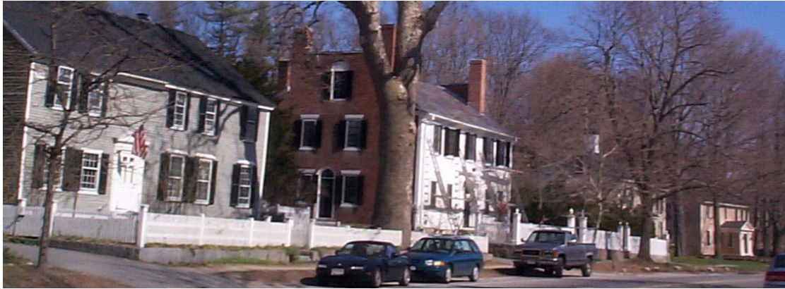
Houses along lower Lexington Road, American Mile Historic District. The Capt. John Adams House, ca. 1817, center, displays the most stylish and well-preserved of any Federal style doorway in Concord.
