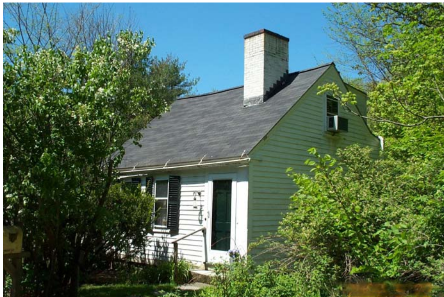
475 Monument Street, J. Monroe (Darby Ferguson House), early 19th C. Monument Square/North Bridge Historic District. Significant as the only one of the town's few early-19th C. 1 1/2 story "half cottages" that has not been greatly enlarged.
