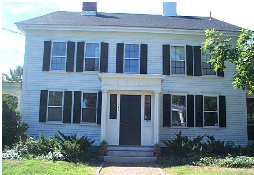
185 Main Street, Prescott/Munroe House, ca. 1810/1844. Main Street Historic District. Although built in the Federal period, it was remodeled in the mid-1840's in the Greek Revival style. The 1827 -35 home of the John Thoreau family as tenants, including Henry Thoreau who was ten upon moving in. Bought in 1844 by William Munroe, Sr., best known today as the inventor of the first American-made lead pencils, an industry taken up by several others in the Concord area including the Thoreaus.
