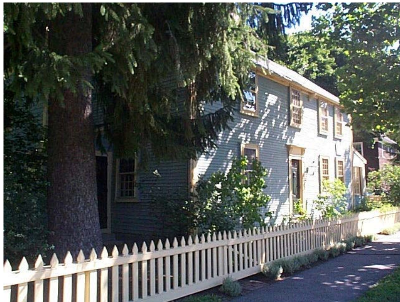
Benjamin Barron House, 245/249 Lexington Road, ca. 1716. Built by Benjamin Barron, the owner of Concord’s best-known slave, John Jack, who bought his freedom. The ca. 1716 house is a First Period 2 1/2 story, 1-room-deep center-chimney structure with an asymmetrical 4-bay façade. Together with 255 Lexington Road this is a rare survivor of a house/shop arrangement once prevalent along Lexington Road.
