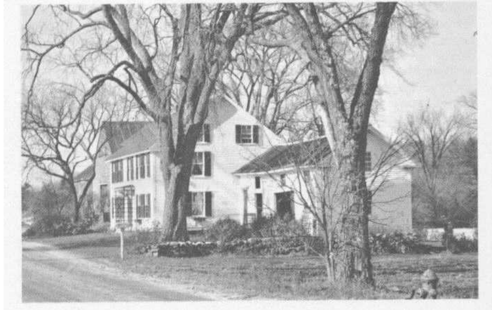
448 Barrett's Mill Road, Colonel James Barrett Farm, 1705. Barrett Farm Historic District. Highly significant both as the home of Colonel Barrett, Revolutionary War patriot and commander of the provincials who fought at the North Bridge on April 19, 1775, and as a storehouse for arms and supplies. Photograph circa 1958.
